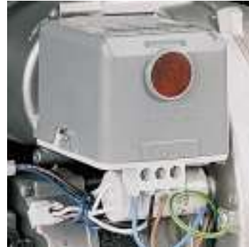
Control box fitted with an ignition transformer
